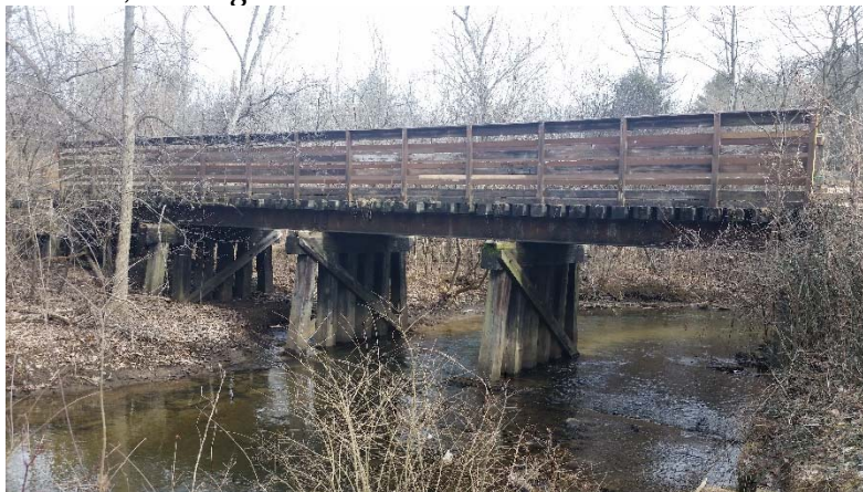
Bridge 33.7 – Span over Paint Creek. Taken from the west looking east
