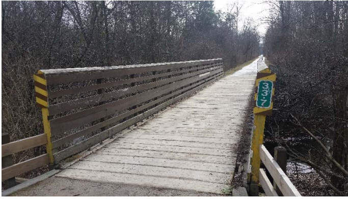
Top of bridge. Taken from the north side, looking south.
